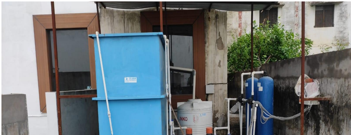
Sewage Treatment Plant
