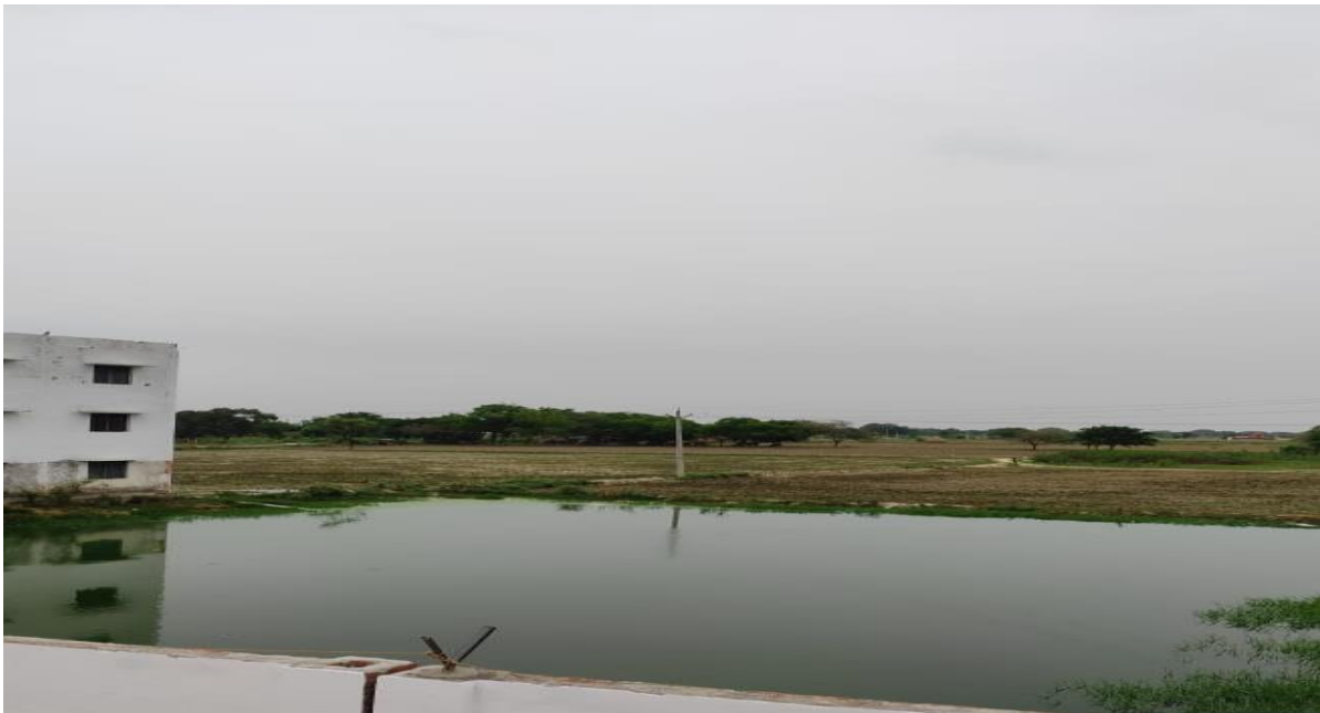
Pond for storage of Waste/Harvested Water
