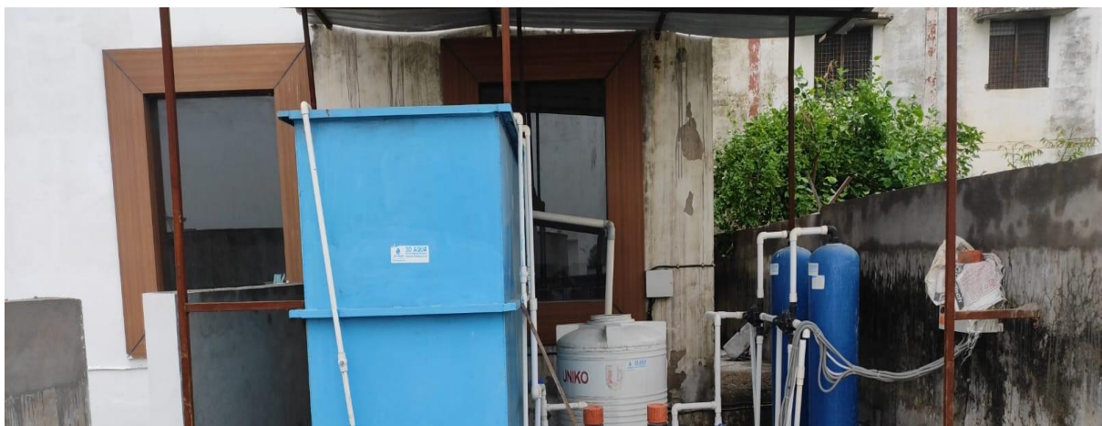
Sewage Treatment Plant
