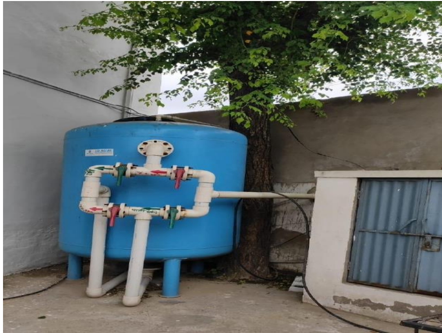
Water Treatment Plant
